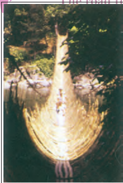
Figure 6.7 : Rope Bridge (Arunachal Pradesh)
