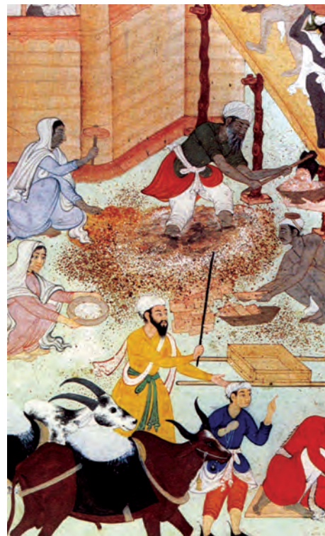
Fig. 8.8 a The construction of Fatehpur Sikri – women crushing stones
