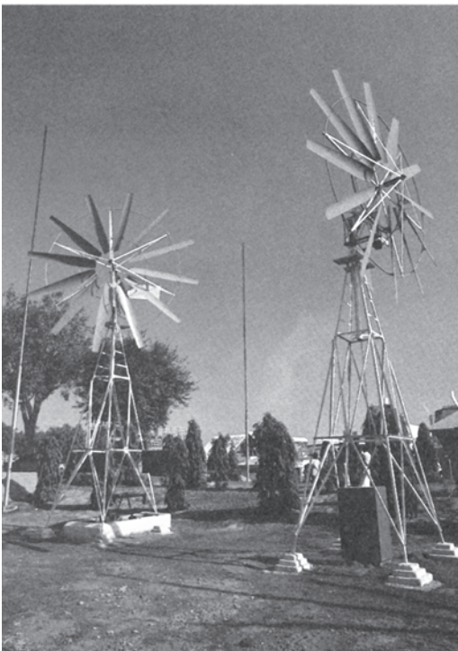
Fig. 8.7 Wind mill : another source of generating power
