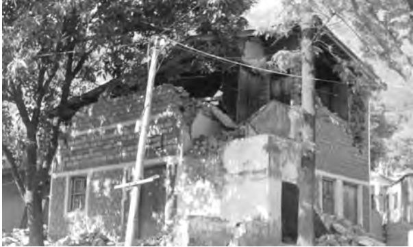
Figure 7.1 : A Damaged Building Due to an Earthquake
