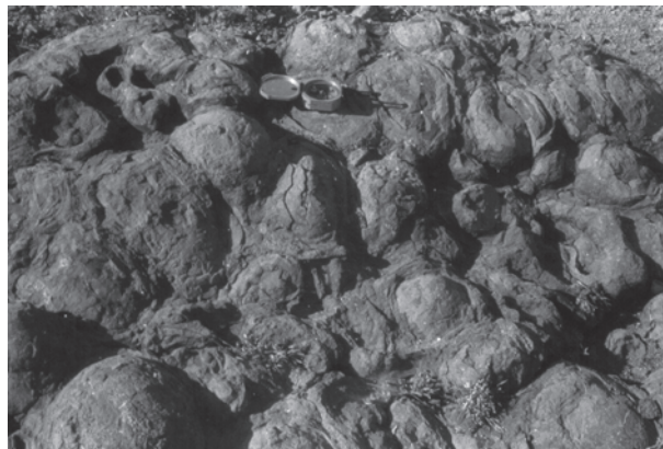
Fig.6.4 : Exfoliation (Flaking) and granular disintegration
